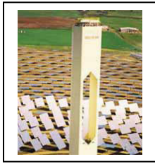
Figure 6- Power Tower technology demonstrated by PS-10 project in Spain
