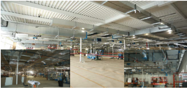
Fig. 4. Installation of HVAC equipment
