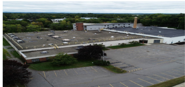
Fig. 2. Pittsfield facility prior to demolition
