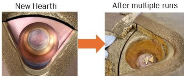
Fig. 2. Excessive metal buildup on the hearth pocket due to Au wicking out of the liner.
